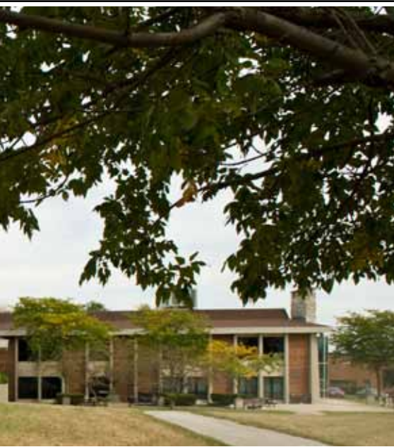
Above: The exterior view of James F. Dicke Hall; the glass facade offers a full view of beautiful Grand Lake St. Marys.
